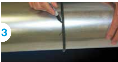
3 Use O-ring provided and mark for cut.
