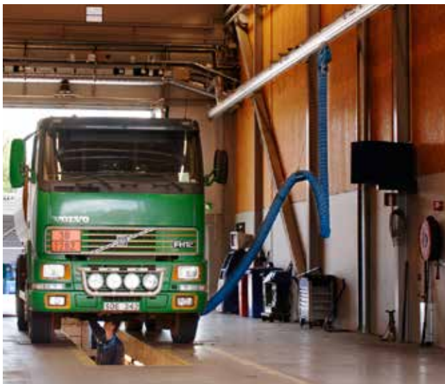
Example exhaust system for vehicle inspection.
