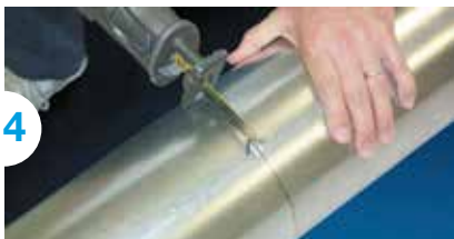
4 Cut the duct.
